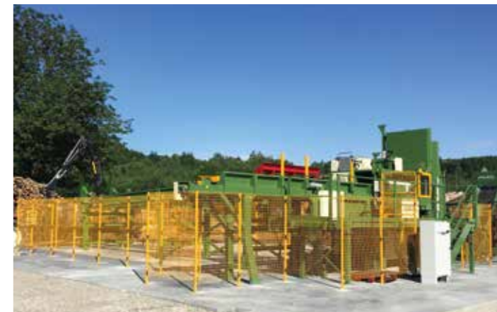
Safety barriers to delimitate the working area
